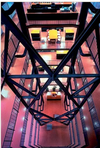
ArcelorMittal office building (AOB), Luxembourg
