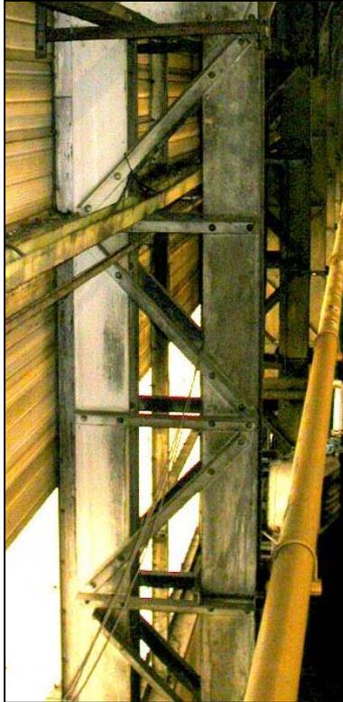
**Figure 2.4 Built-up column with lacings in an industrial building**
