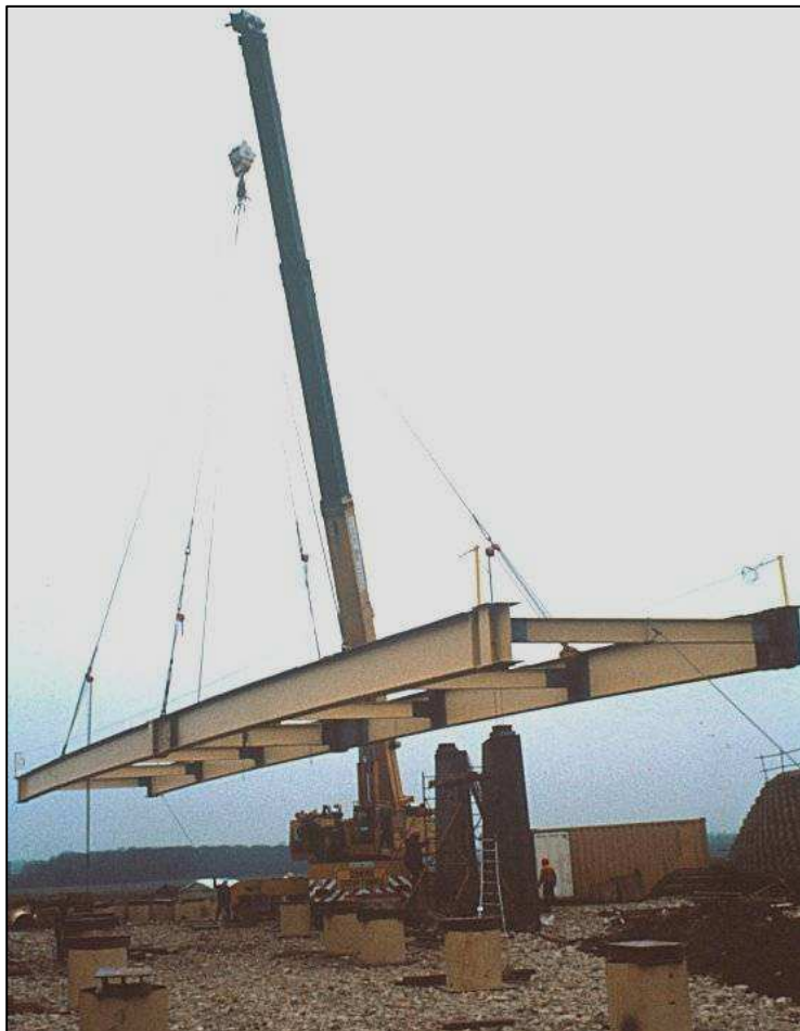
Preassembled steelwork (35t) lifted into position
