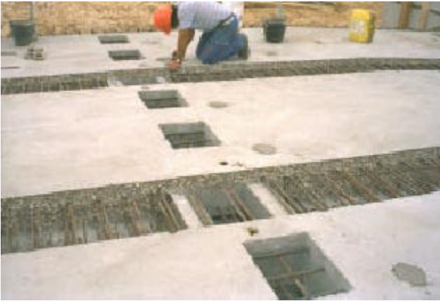
Figure 4-49: Prefabricated slab. Example of transverse joint detailing:
