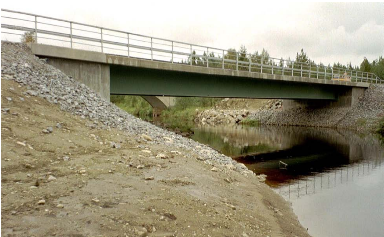
Figure 4-3: Bridge with integral abutments.
