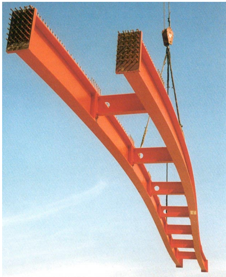
Figure 4-36: Main girders with thick cap plates and studs
