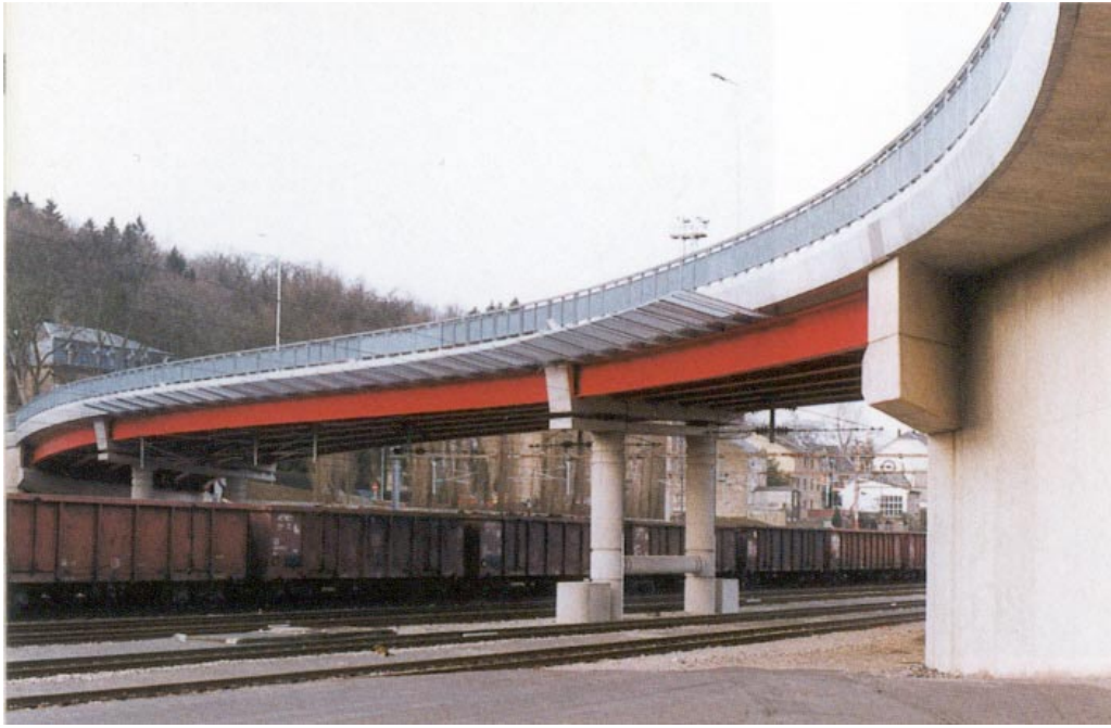
Figure 4-35: Three span bridge in Differdange
