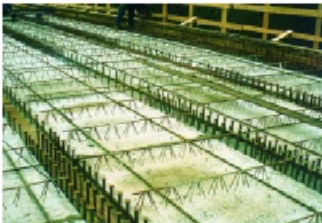
Figure 4-47: Precast reinforced concrete panels used for permanent formwork.
