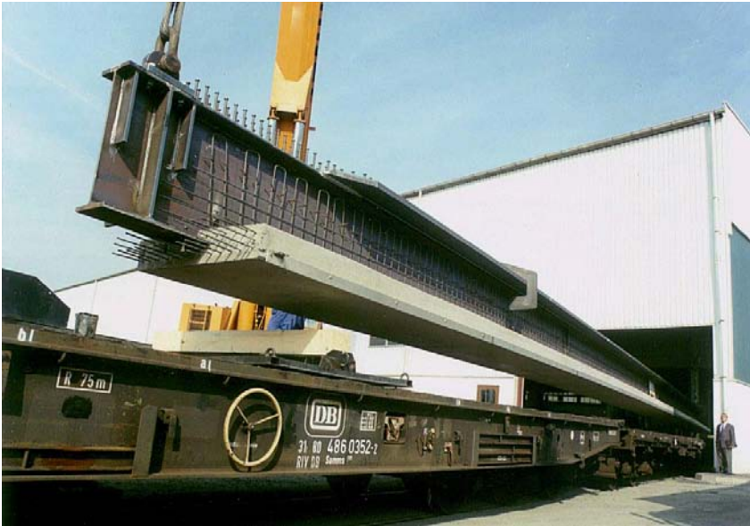
Figure 4-52: Transportation of a Preflex beam
