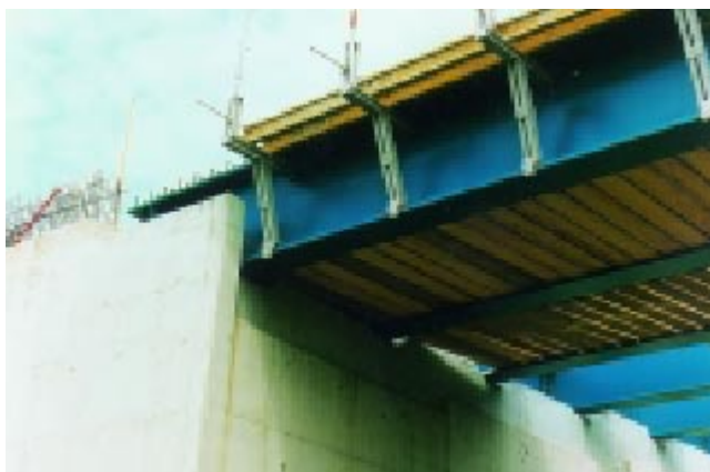
Figure 4-48: Example of formwork support for cantilever part of slab.
