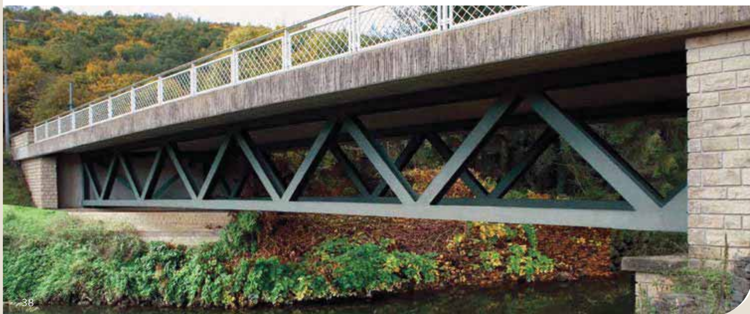
Bridge over the Alzette river in Cruchten, Luxembourg – Transparent truss structure in composite action without gusset plates – S460 rolled steel sections have been used as truss members.
