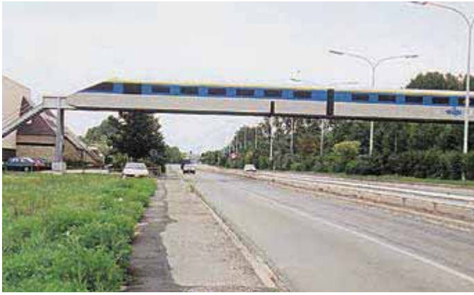
Footbridge for the visitors of a leisure park in Wavre, Belgium – Through type bridge with thematic enclosure.
