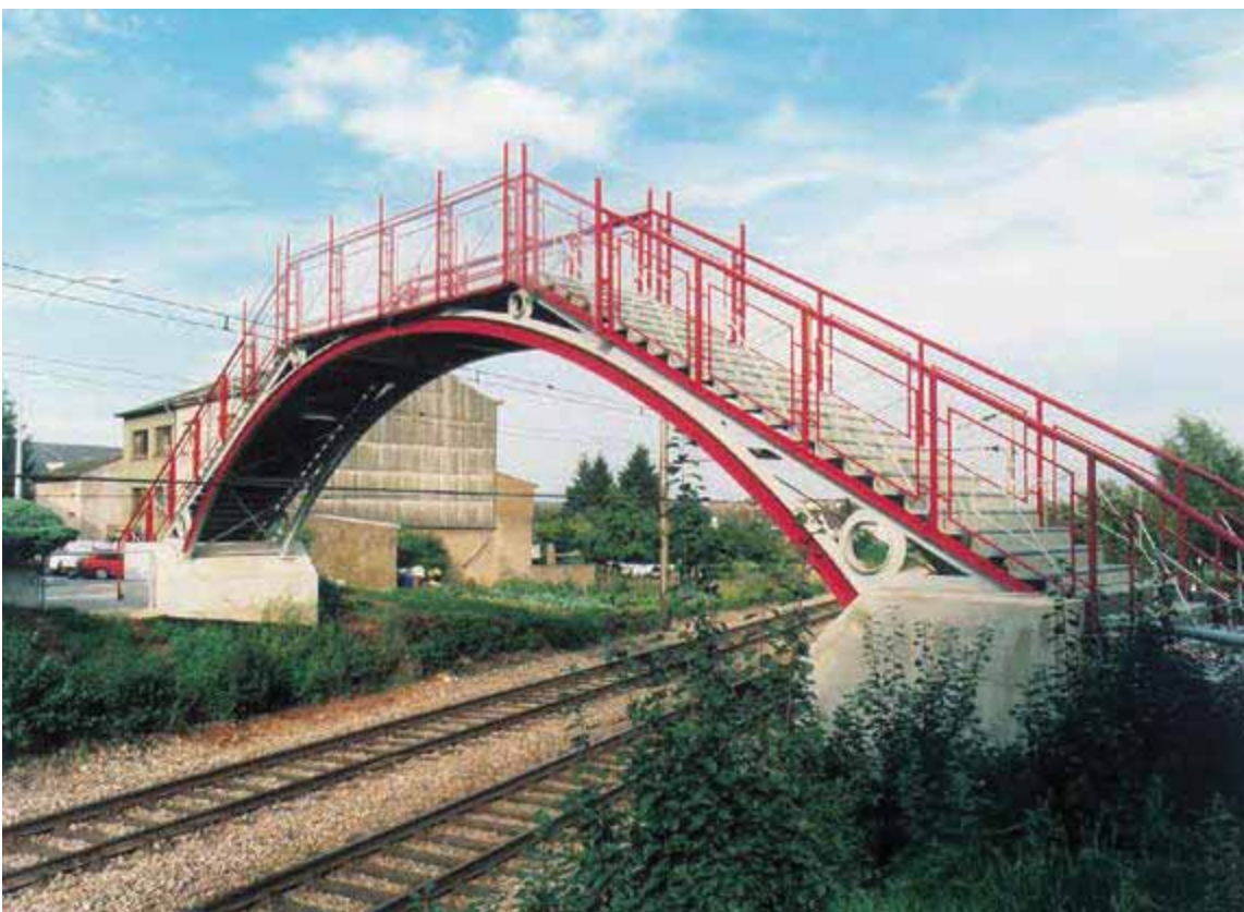
Footbridge near Schifflange, Luxembourg – Principle beams with an extreme curvature.
