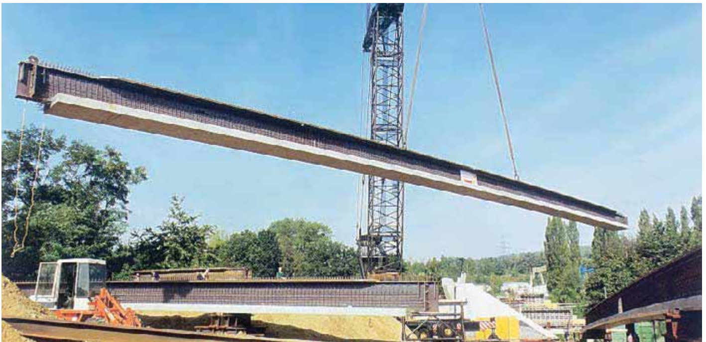
Single span bridge in Kerpen Horrem, Germany – 41.25 m long HE 1000 A beams used for prestressed composite girders of “Preflex” type.
