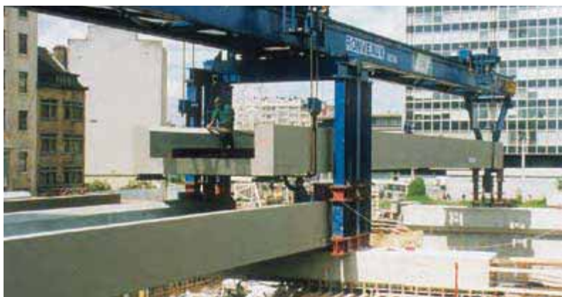
Extension of the Brussels - South Station for the Eurostar trains - A launching gantry is used for fast erection of prefabricated prestressed composite decks.
