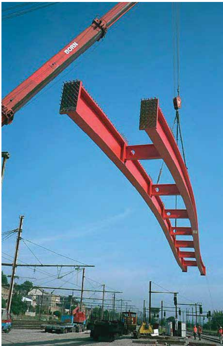
Road bridge in Differdange, Luxembourg – Erection of two main girders of a composite bridge by crane. The rolled girders are curved along both cross-sectional axes in order to adapt them to the geometry of the road.
