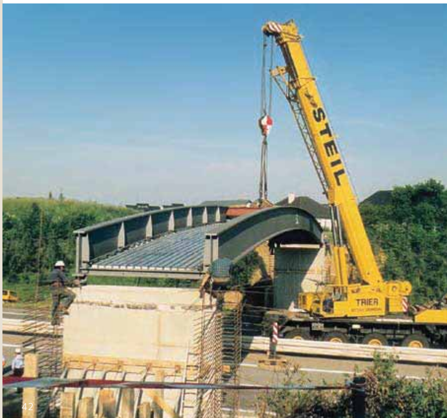
Erection of half-through type structure – Pre-assembled framework including permanent steel shuttering is lifted into position by crane.
