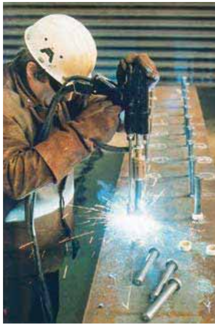
Finishing workshop - Welding of shear stud connectors.
