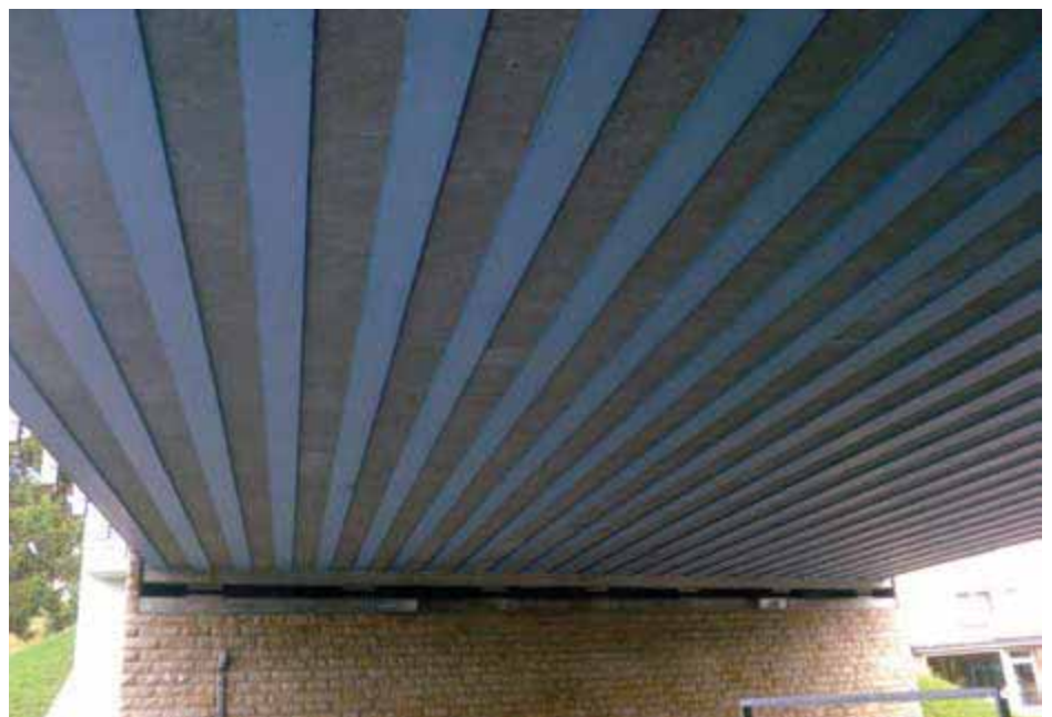
Lower side of a filler beam deck – Only the bottom flanges of beams are visible.
