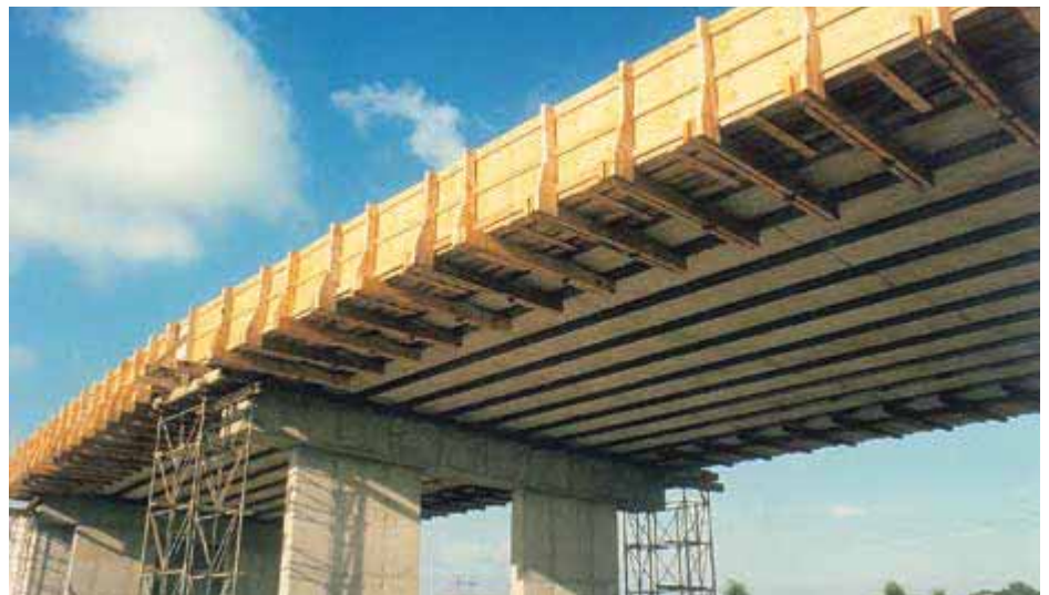
Construction of an overbridge of A104 motorway, France – Falsework is not required. Disruption of motorway traffic is minimal.
