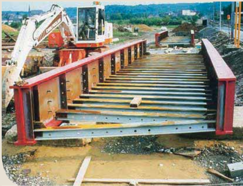
Railway bridge over the Emile Mark street in Differdange, Luxembourg – The replacement of an old deck with direct track fastening by a ballasted track bridge required a structural system with minimized construction depth. A half-through girder deck solved the problem. The picture shows the assembled steel framework before concreting.
