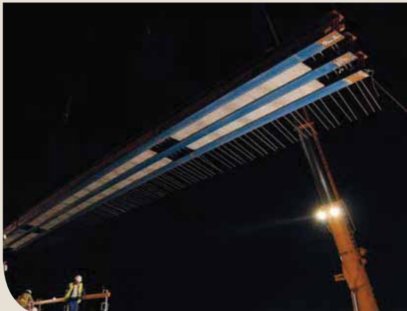
Railway bridge at Sète-Frontignan, France - Lifting in of a pre-assembled part over an existing railway line.
