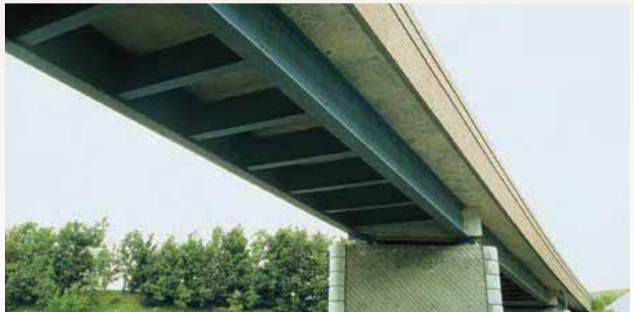
Railway bridge over the A23 motorway in Fretin, France – Four-span bridge with spans of 16.9 – 21.9 – 23.0 – 17.8 meters. The two continuous main girders and the bracings within spans are rolled beams; the cross beams at supports are made of reinforced concrete.
