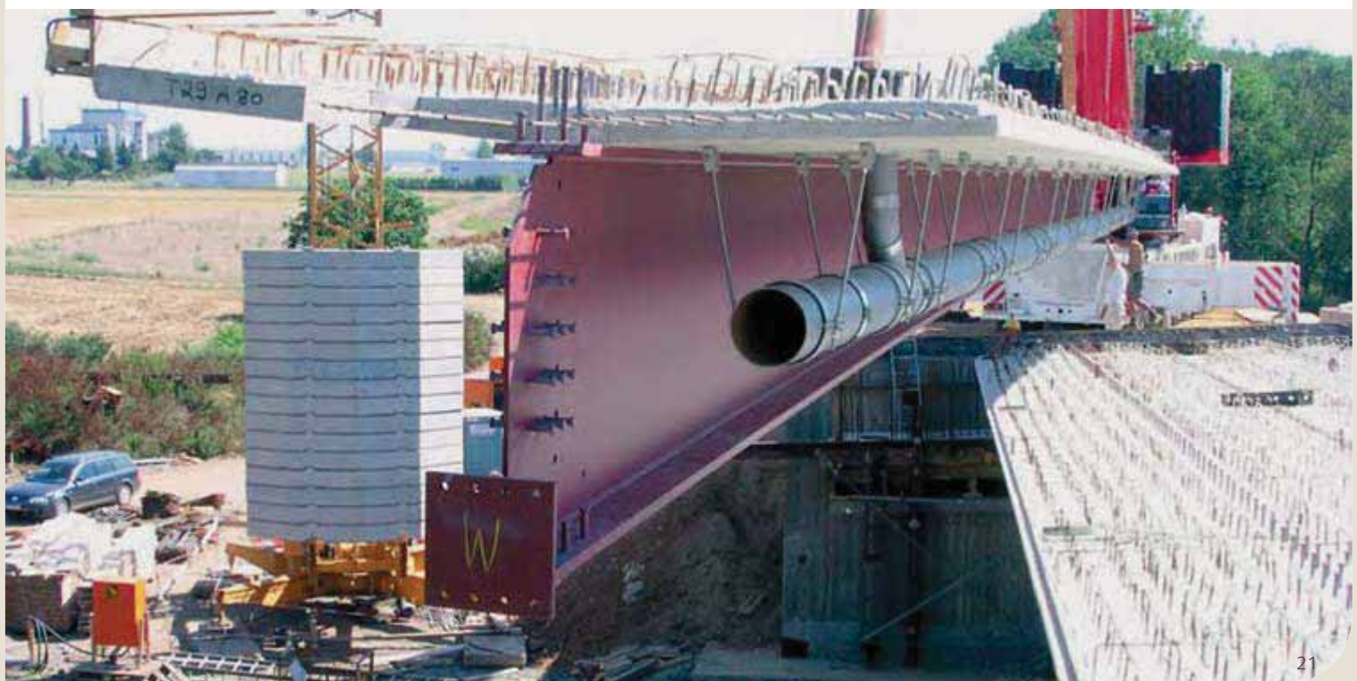
The Horloffthalbridge in Hungen, Germany - Lifting in of a partially prefabricated beam.
