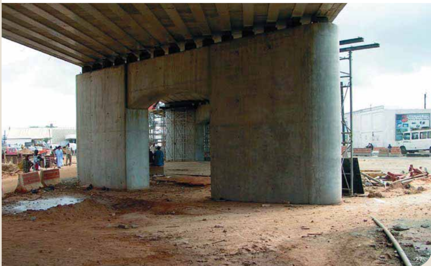
Pont de Cyrnos in Senegal – Bottom view on the filler beam deck and support.
