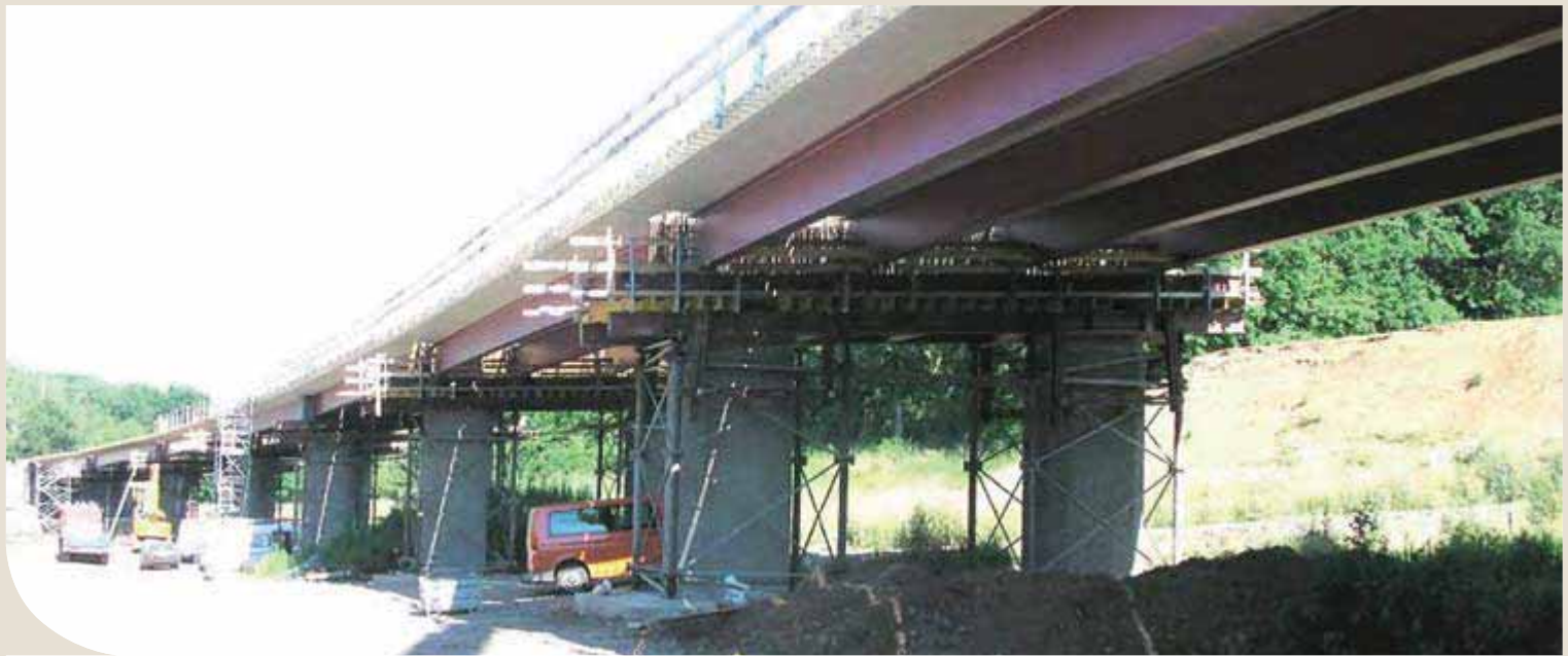
The Horloffthalbridge in Hungen (Germany) with eight spans constructed in 2006. For five spans partially prefabricated concrete beams with heavy rolled beams in S460 have been used.
