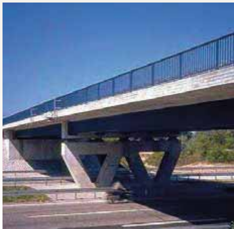
Road bridge in Bremgarten, Germany – With concrete cross beams and indirect support.
