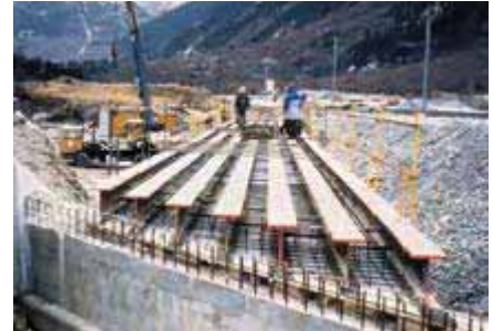
Construction of a filler beam railway bridge as part of the Puymorens road tunnel link between France and Spain.
