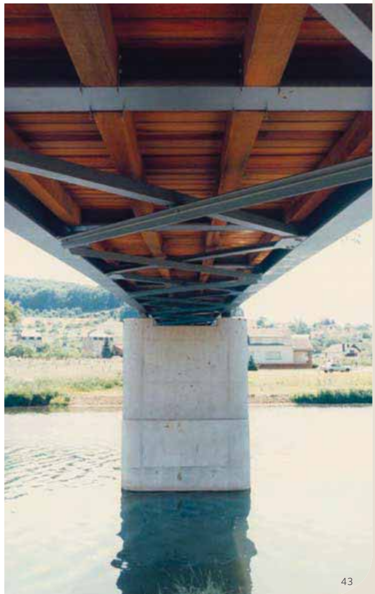
Bottom view on the stiffening elements of the bridge in Steinheim, Luxembourg
