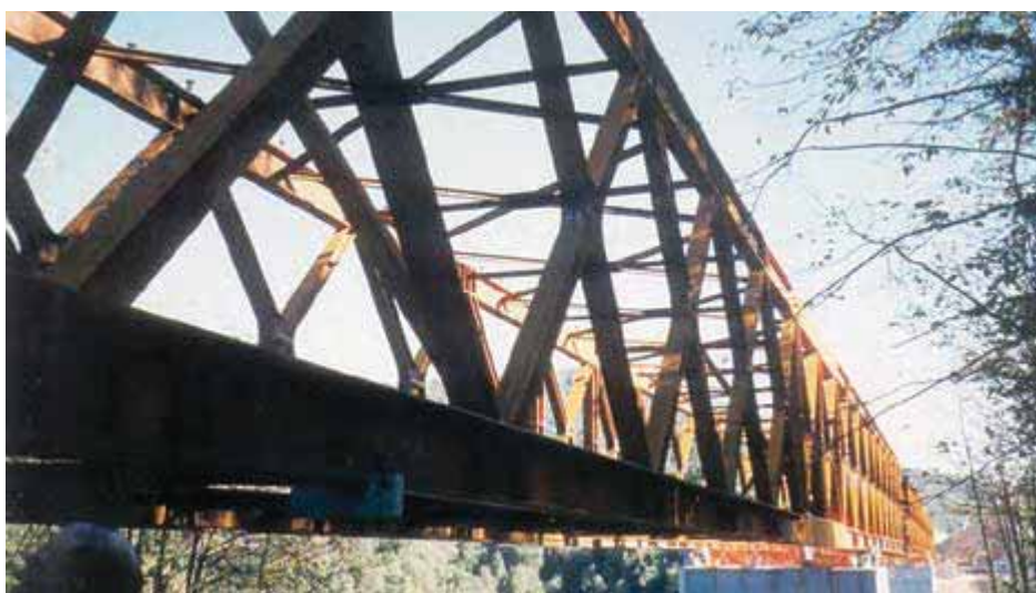
Costa Martina road bridge, Spain – Rolled beam truss girders, continuous over 3 spans of 60.6 – 121.2 – 60.6 m. The picture shows the bridge before the erection of the precast slab elements on the upper chords.
