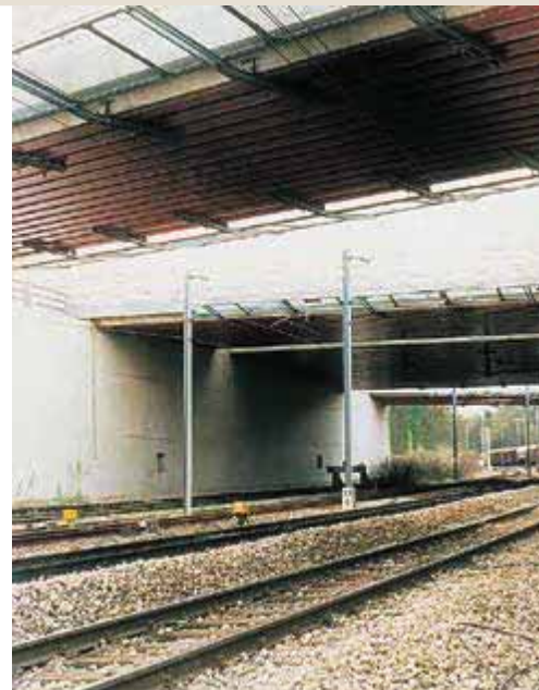
Filler beam bridge built over a heavy traffic railway line – High quality coating provides durable protection to lower flanges.
