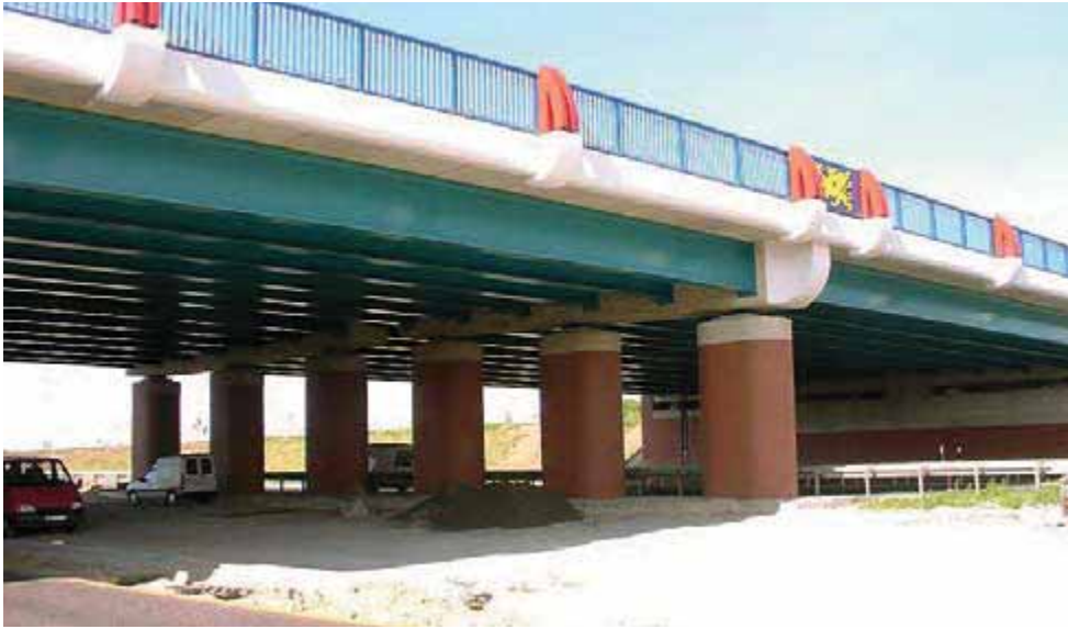
Composite bridge with concrete crossbeams at Bentwisch, Germany – Design combining steel and colour.
