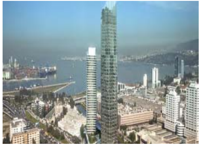
Figure 7.14: Mistral Residential Tower, Izmir, Turkey
