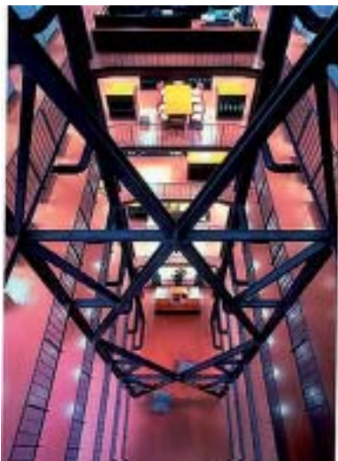
ArcelorMittal office building (AOB), Esch-sur-Alzette, Luxembourg
