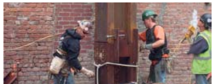
Figure 7.2: Column joint before welding
