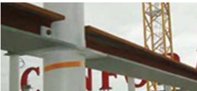
Figure 6.6: Slim-Floor for parking in IFB (Nantes, France)
