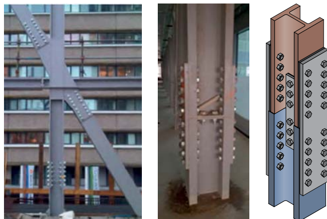
Figure 7.1: Bolted connection of two HD/UC/W columns
