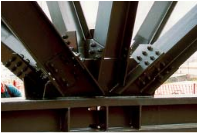
Figure 7.7: Mariner Stadium close up on gusset plates connection in S355 (Gr. 50) with S460 (Gr. 65) beams
