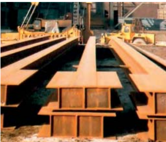
Figure 8.1: Driven piles with reinforcement at the base to increase the cone friction resistance and thus provide support for high loads
