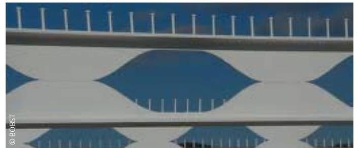
Figure 6.4: Angelina® beams
