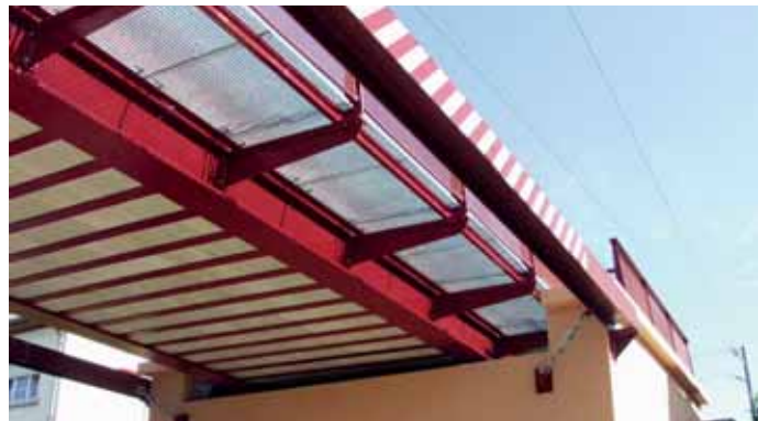
Half-through bridge deck in Dudelange, Luxembourg
