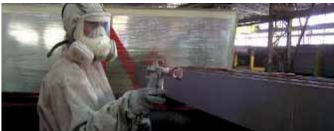
Manual application of an organic layer
