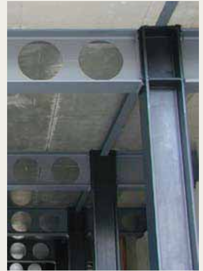
Figure 17 Beam to column connection
