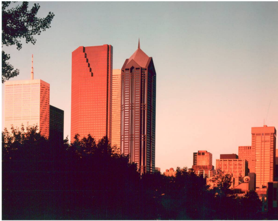
Image courtesy WZMH Architects Figure 2: Bay Adelaide Centre, South Tower (original design)
