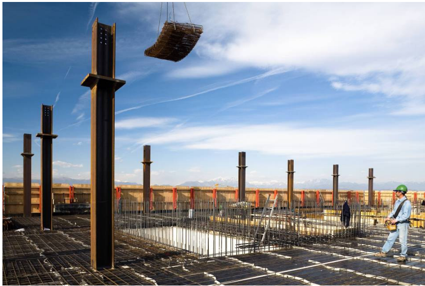
Figure 15 Slab under construction, © Arup
