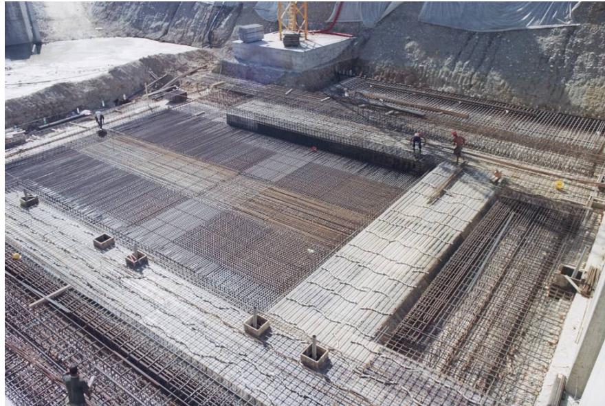
Figure 22 Raft foundation reinforcement, © Arup
