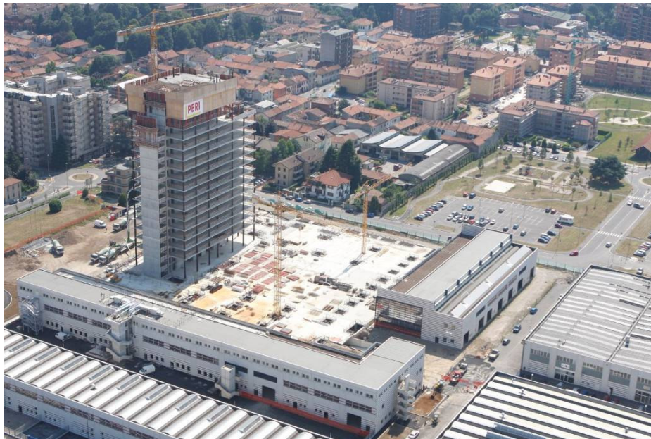
Figure 3 Intermediate levels under construction, © Addamiano Engineering
