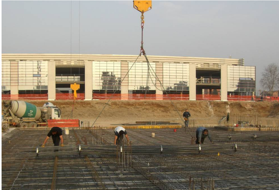
Figure 16 Flat slabs – Bamtec technology, © Arup
