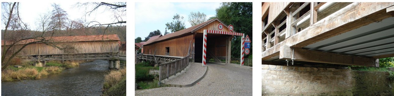
Fig. 4 Landmarked wooden bridge in Buchfart, Germany, after deck replacement
