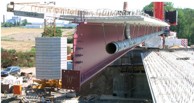
Fig. 1 Horlofftal Bridge: Placing of the prefabricated composite beams
