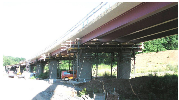
Fig. 2 Horlofftal Bridge: Almost finished bridge
