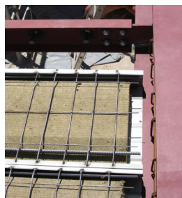
Fig. 2: EPL – SFB and Cofradal
