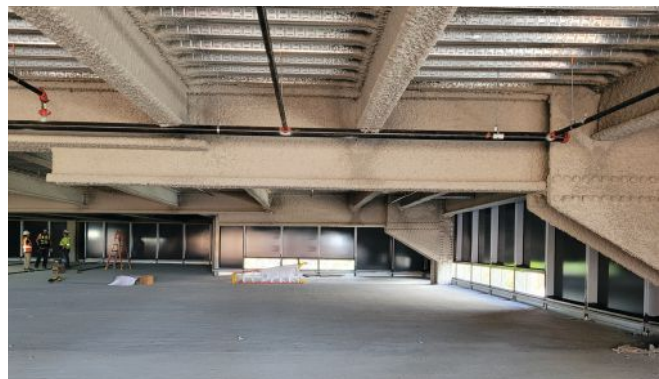
above and below: Two views of the cut-out portion of the transfer truss, which was designed to alleviate a low head height condition without having to adjust the floor-to-floor height at the level under the transfer truss.
