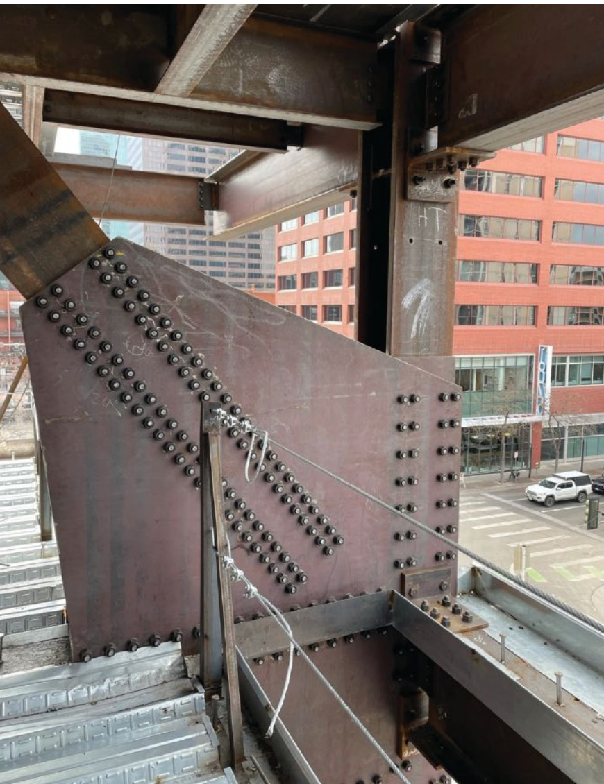
below: The actual bolted connections.
