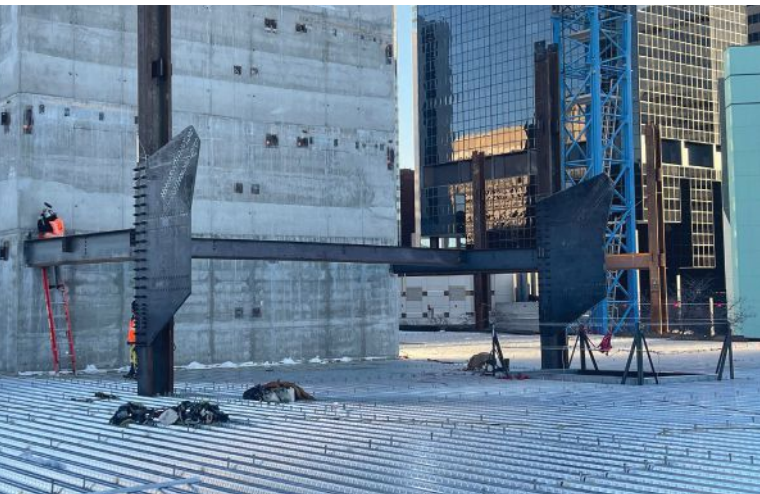
below: Steel framing attaching to the concrete core.
