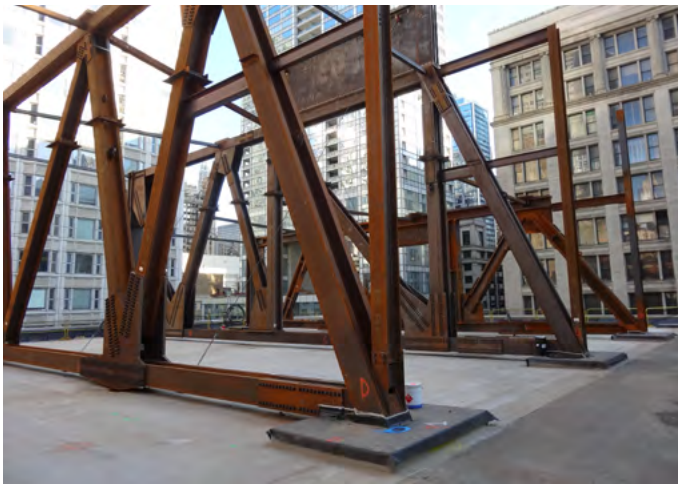
A913 Grade 65 sections used in transfer trusses
