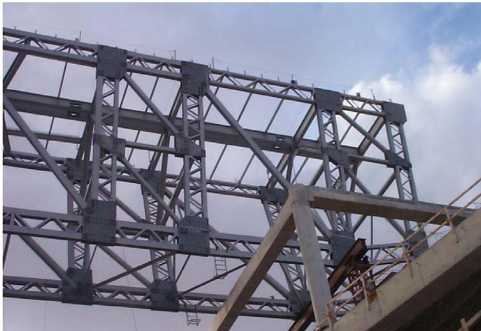
*Figure 4: Typical Bay of Supertruss*
