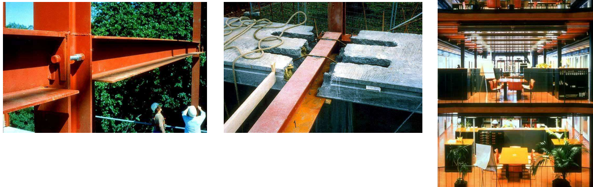
Figure 1: Office building in Esch-sur-Alzette, Luxembourg [1]
