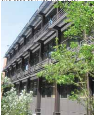
Office Building, Esch/Alzette (L)
