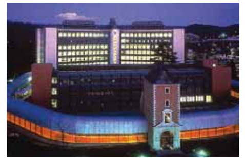
ArcelorMittal Head Office at Esch-sur-Alzette, Luxembourg
