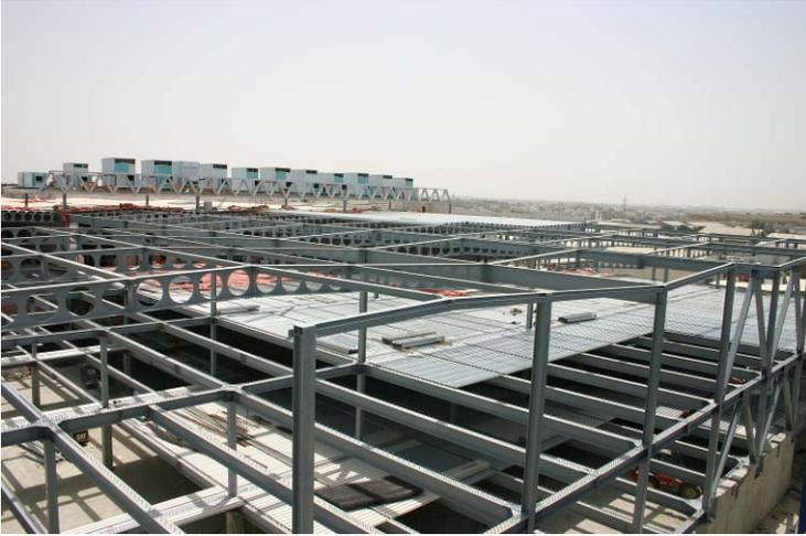
figure 3 – The composite steel-concrete floor with column at 8.00 by 16.00 m centres, main and secondary beams continuous
