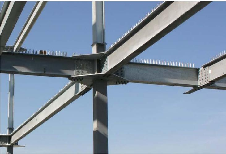
figure 4 – The two way beam to column moment resisting connection
