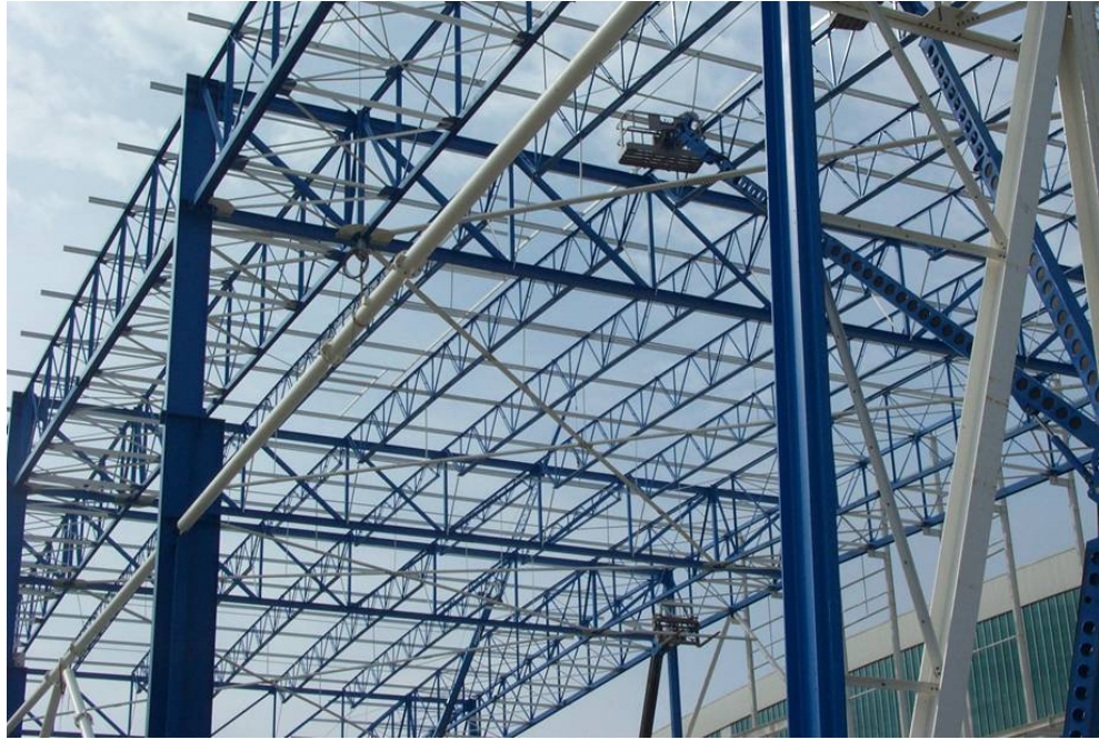
Figure 1.7 N-truss (also with N-truss purlins)
