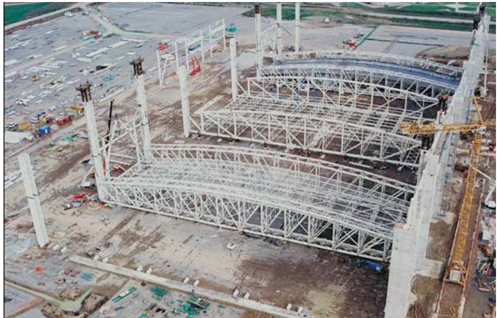
Figure 1.6 N-truss – 100 m span
